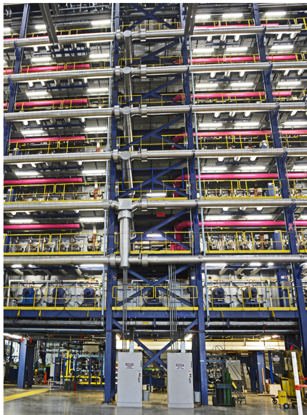
The new hot dip galvanizing line that AK Steel has installed at its Dearborn Works
