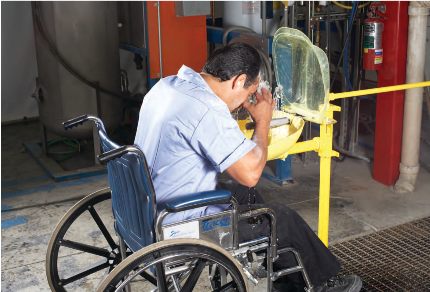
In addition to being accessible from any direction, eyewash stations should be handicap accessible.
