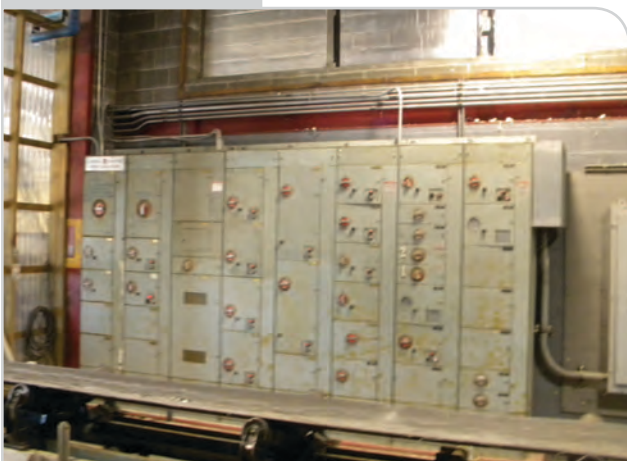
View of motor control center.
