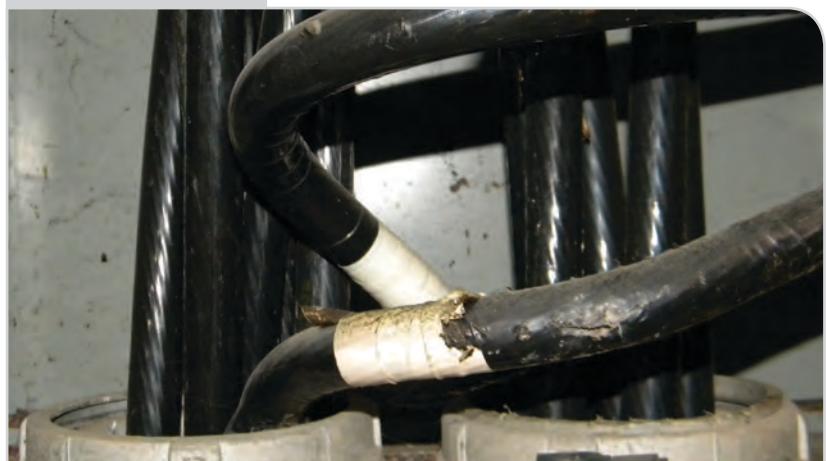
View of cables and conduit.
