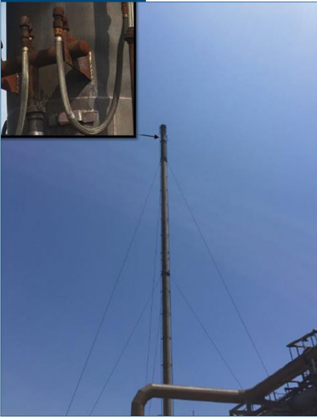
A UAV was used to inspect pilot burner piping connections on the flare stack of a byproduct plant at Stelco.
