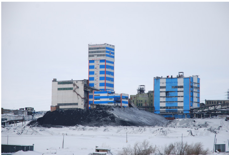
Vorkutinskaya mine in Russia, the first of Vorkutaugol's mines that was equipped with the modern gas analytical system Mikon-3. Photo courtesy of Severstal.
