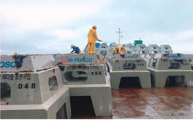
POSCO Triton blocks are planted with marine algae ahead of being installed on the sea bed.
