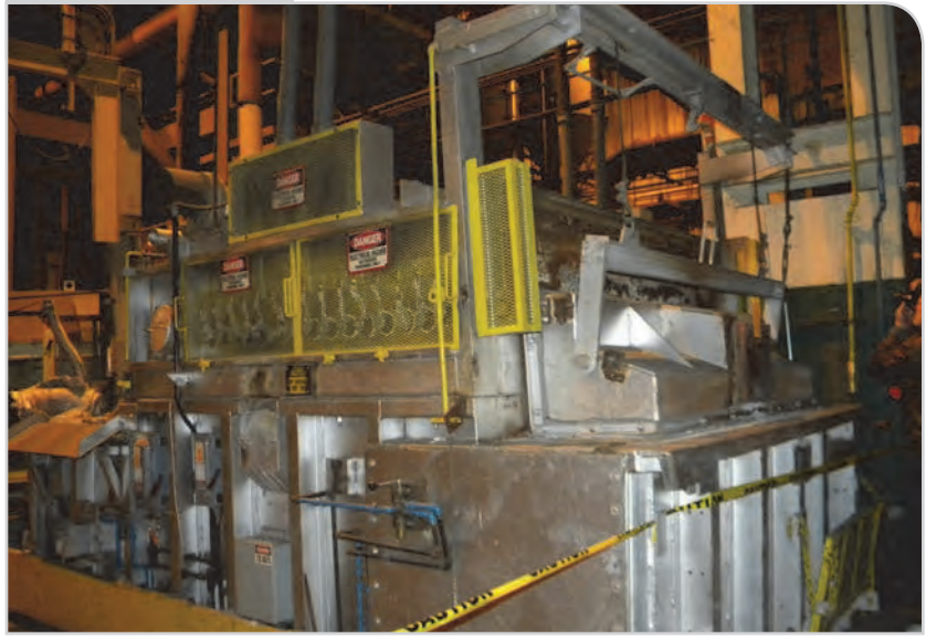
Rebuilt furnace and footed door.
