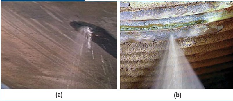
Leak in a non-pressurized spray cooling system (a) vs. leak in a pressurized tubular system (b) (5 gallons/hour vs. 16,000 gallons/hour).
