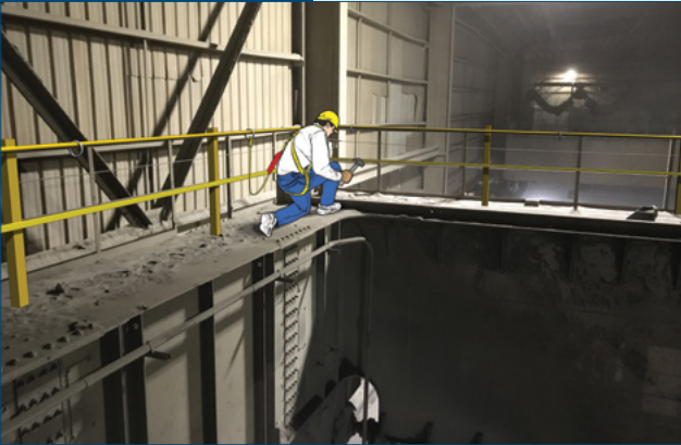
Conceptual design of a fall protection solution for bridge crane and end trucks.
