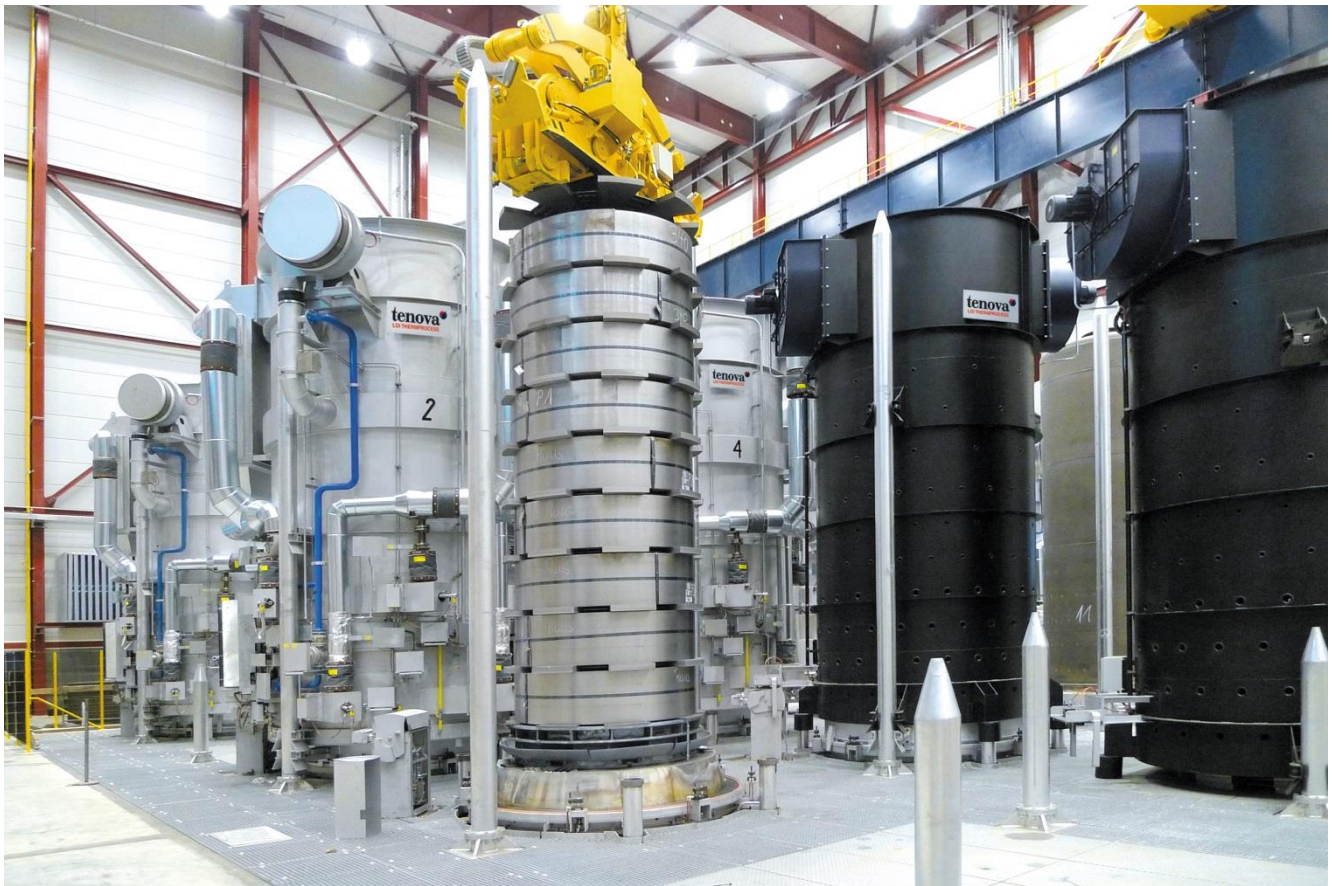
Fig. 1: Tenova LOI Bell-type Annealing Plant with Fully Automatic Crane Operation in the works of BILSTEIN, Hagen-Hohenlimburg, Germany
