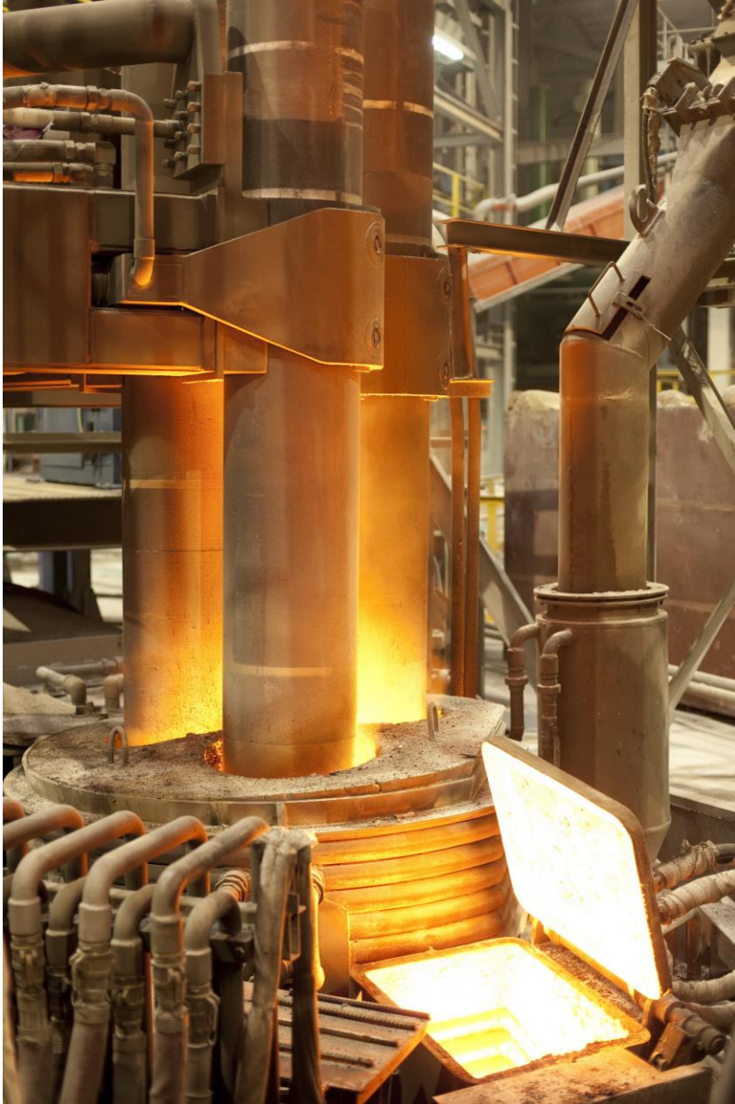
ArcelorMittal Temirtau receives a new 290-ton ladle furnace from SMS group.
