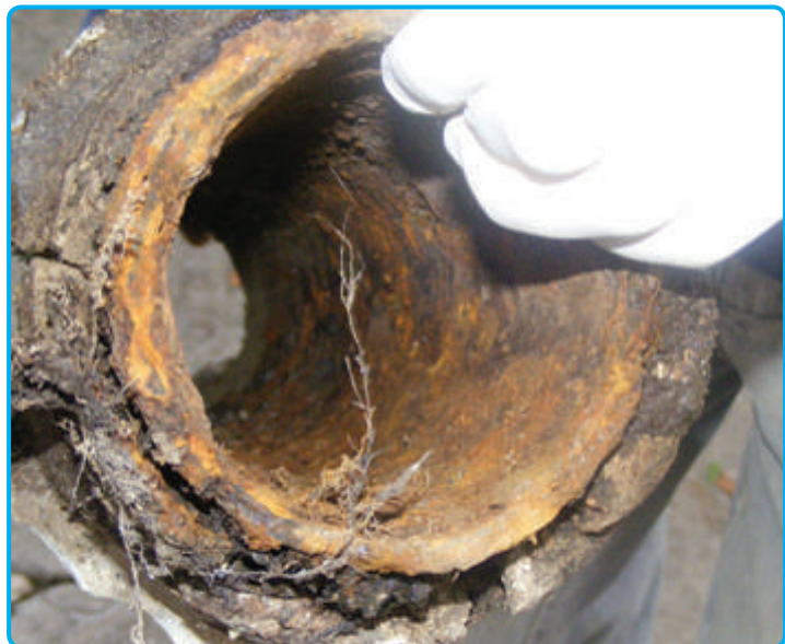
Fig.(1): The corrosion of metallic pipe.
