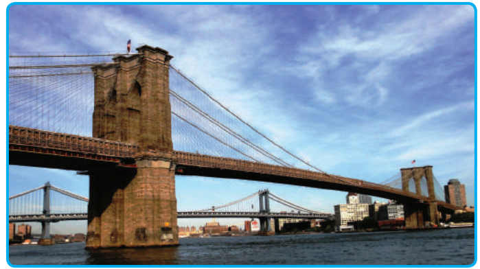
Fig.(3): Brooklyn Bridge
