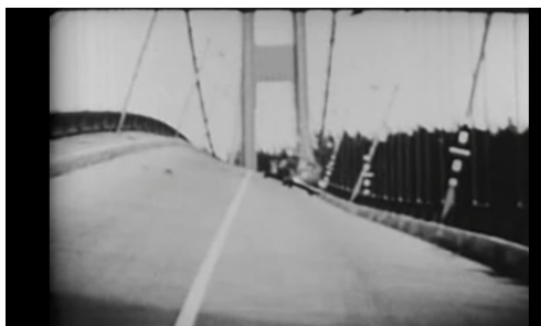
Figure 1 - historic failure of the Tacoma Narrows bridge due to resonance
