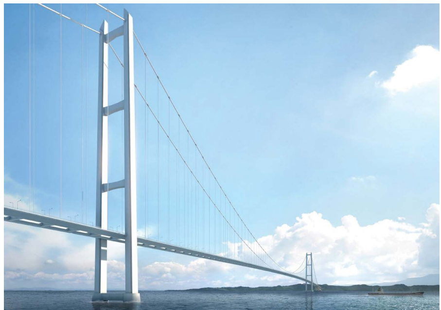
With the span between its two towers sitting at 2,023 m, the Canakkale 1915 is set to become the world’s longest suspension bridge.
