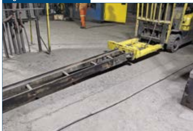
Track installation attachment.
