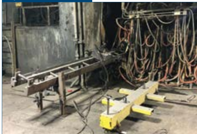
Complete withdrawal straightener track assembled with crawler and roll spreader bar.
