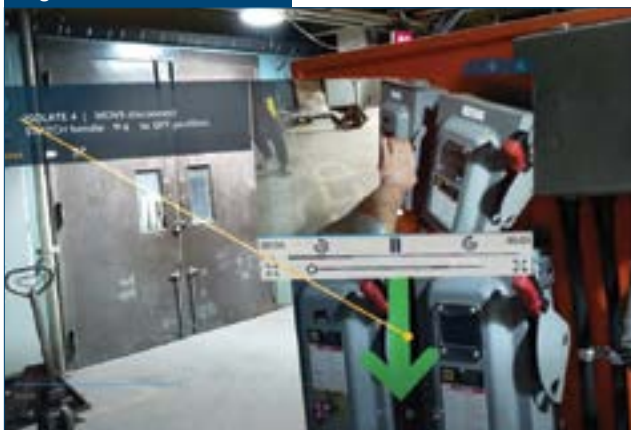
A first-person, user’s view of AR through a stereoscopic AR-enabled head-mounted display i.e., “AR goggles.”
